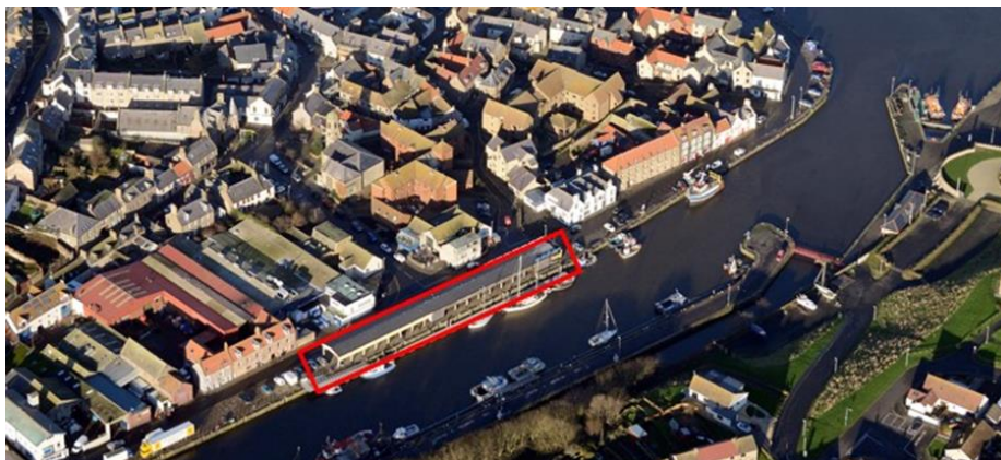
Project site showing the old fishmarket building, demolished in Feb 2021.
