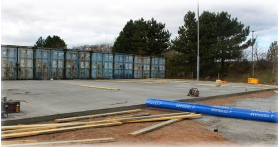
The new fishermen's storage yard – work in progress
