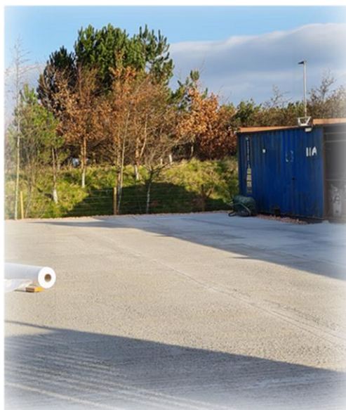
The completed fishermen's storage yard at Gunsreen Industrial Estate
