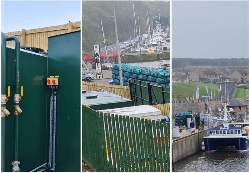
New Fuel and Waste Reception Facilities on Gunsreen Quay
