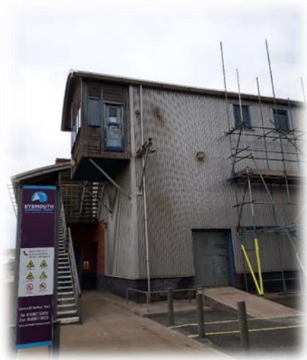
Work in progress, early 2019
