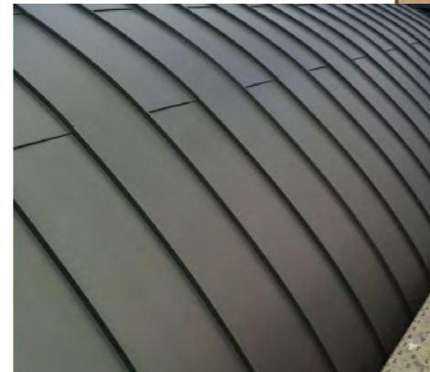
ROOF - ZINC Budgeted Dark zinc roof with standing seams.
