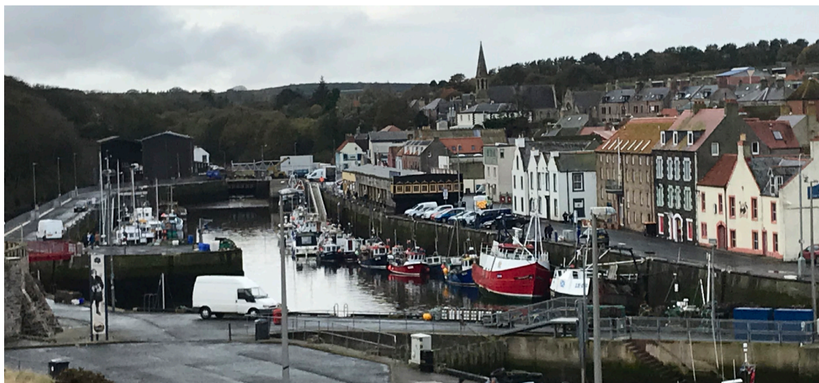
View of the existing Fishmarket Building from Gunsreen House.
